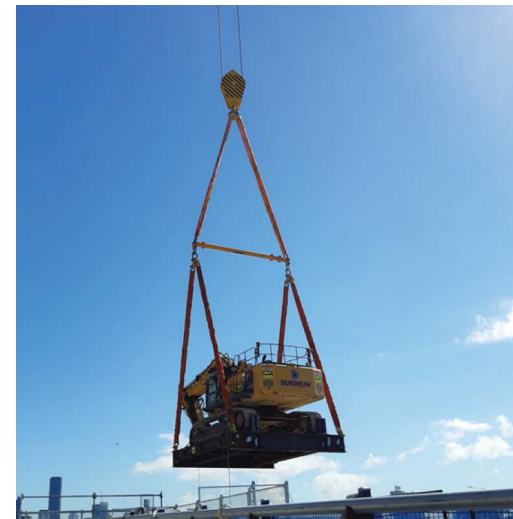
An engineered lifting platform for a 60t excavator.
